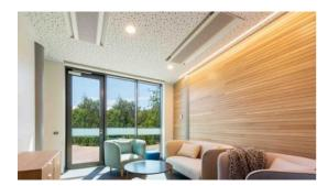
Today, air-water systems are used in many modern buildings and especially in office and administration buildings, offer energy-efficient solutions for the internal space ventilation and air conditioning. There is a variety of installation possibilities for air-water systems, which mean that, for almost every building, variants that meet the most demanding architectural requirements are available.
